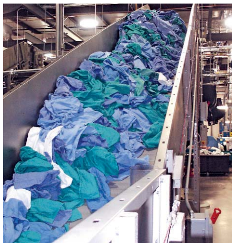
The clean take-away conveyor transports goods from the dryers.
