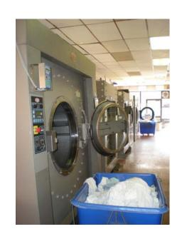
The installed laundry equipment is: one 48040 F7J suspended open-pocket washer-extractor (275 lb. capacity), two 42032 X7J washer-extractors (165 lb. capacity each), one 30022 V6J rigid mount washer-extractor (60 lb. capacity), and three M170
